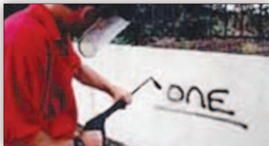
Graffiti cleaning contractor
